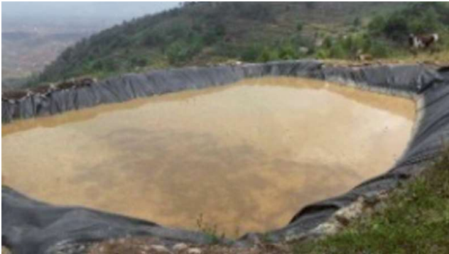
Dam with liner and water collected
