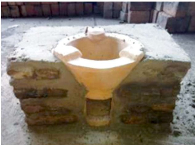
Improved fireplace recessed in fired brick masonry to improve its durability in workability
