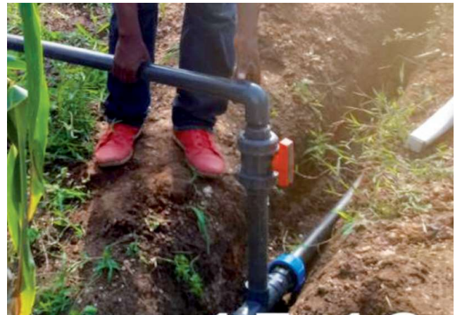
PVC pipe installation for water transport
