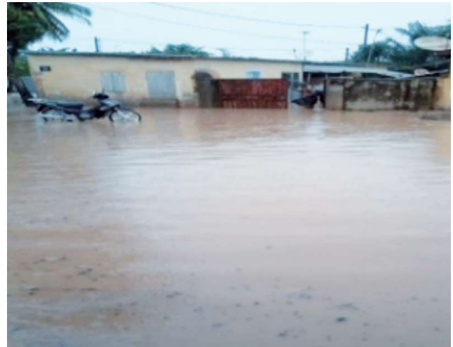
Damage caused by flooding
